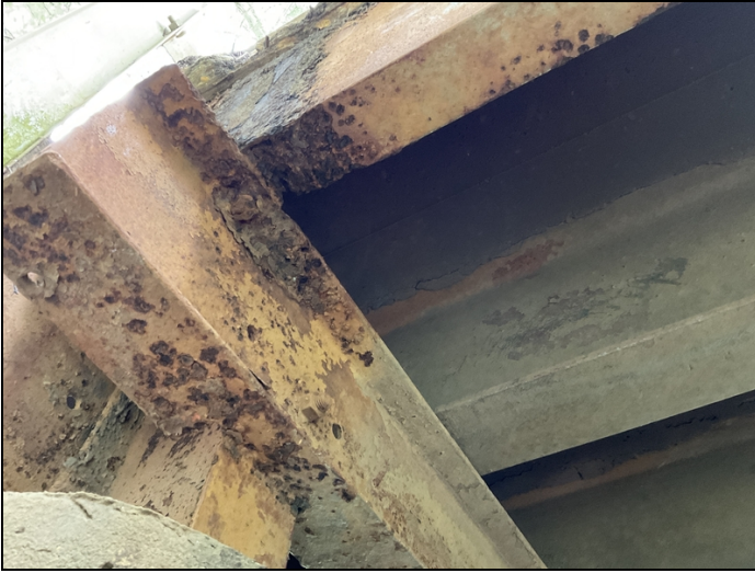
Span 4, Beam 12, Bt 3, hole in bottom flange.
