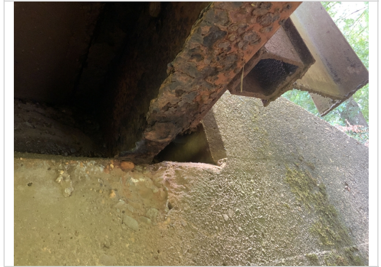
Bent 5 girder 12 section loss at bearing with hole in the web.
