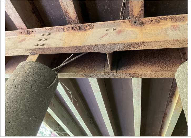
Bt. 3 steel cap, corrosion with minor pitting between columns 2 & 3.
