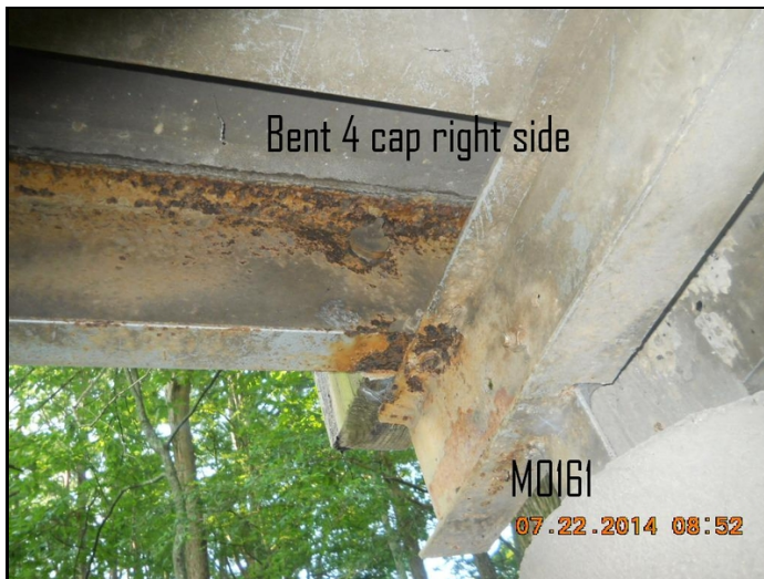
Bent 4 cap rt. side, top flange has some rust with pitting and minor section loss.
