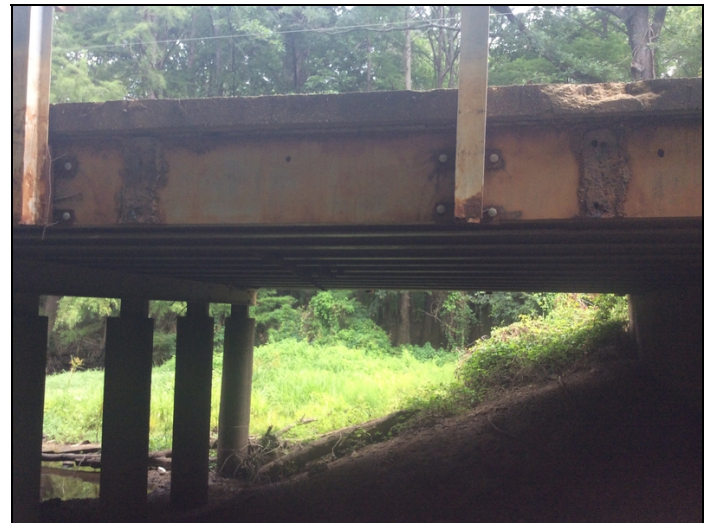
Span 4 Girder 12, there are plates that were welded to outside of girder 12 all spans & appears the old guard rail posts were mounted to these plates. These plates have heavy pack rust and the rust is starting to affect the bottom flange of outside girders @ all locations of the plates.
