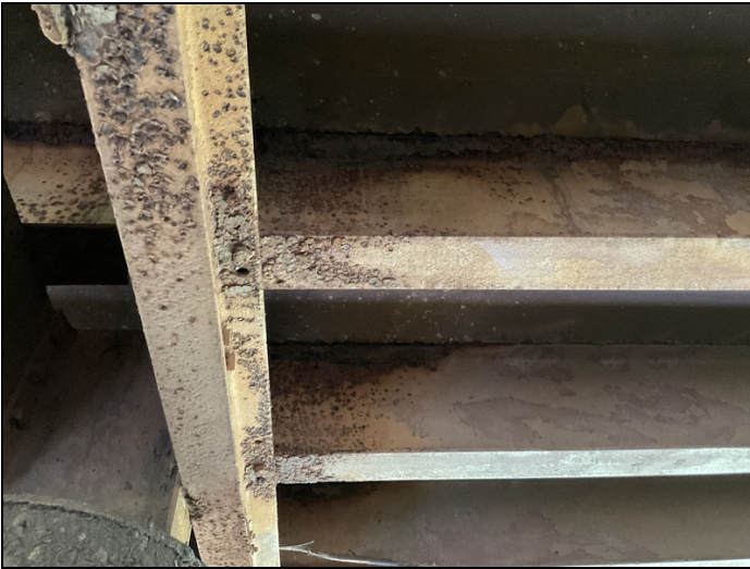
Span 3 at Bt 3, Beams 5 & 6, beam ends have active corrosion with pitting.
