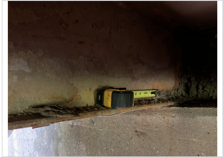
Span 1, Bt. 1, Bm 11, lower web and bottom flange have corrosion with up to 1/4" deep
