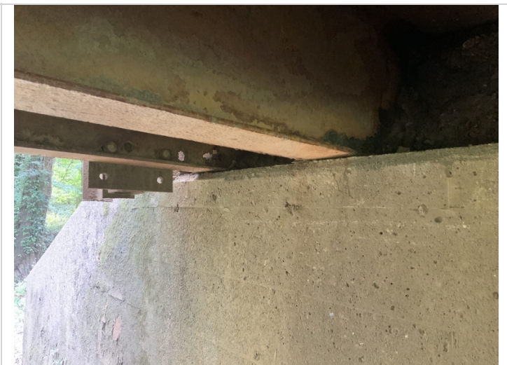
Bent 1 girders 11/12 have holes in web at bearing.
