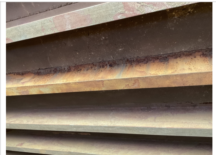
Beam 6, top flange has corrosion the entire length.
